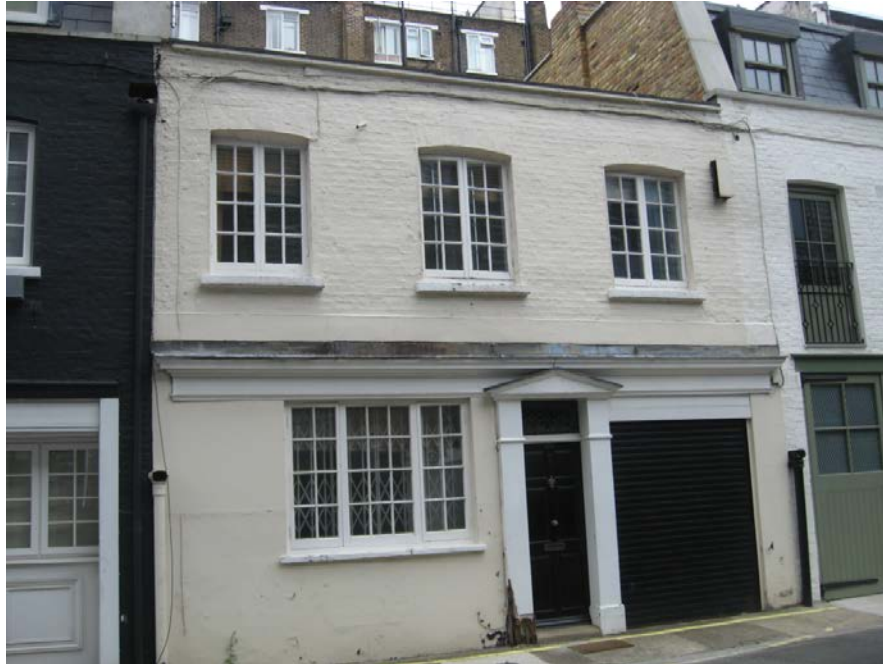
Application site, 103 Eastbourne Mews, front elevation
